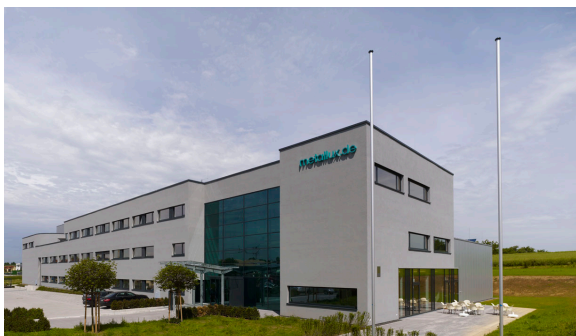
Metallux AG company building in Nellmersbach
